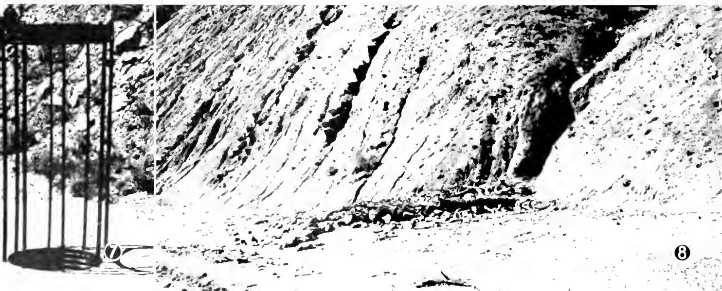
FIGURE 7. Metal debris riser placed over culvert entrance in debris basin. Note provision for extension when debris basin has filled to such an extent as to cause deposition of most of the detritus before it reaches the riser.
